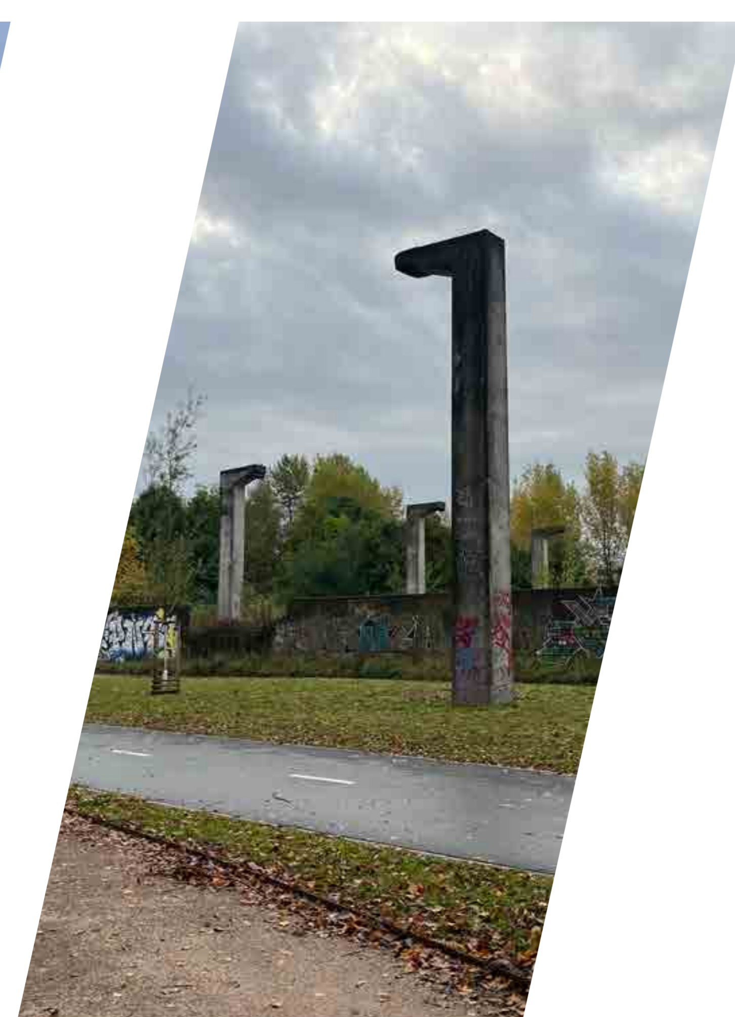
Columns along the crane track.
