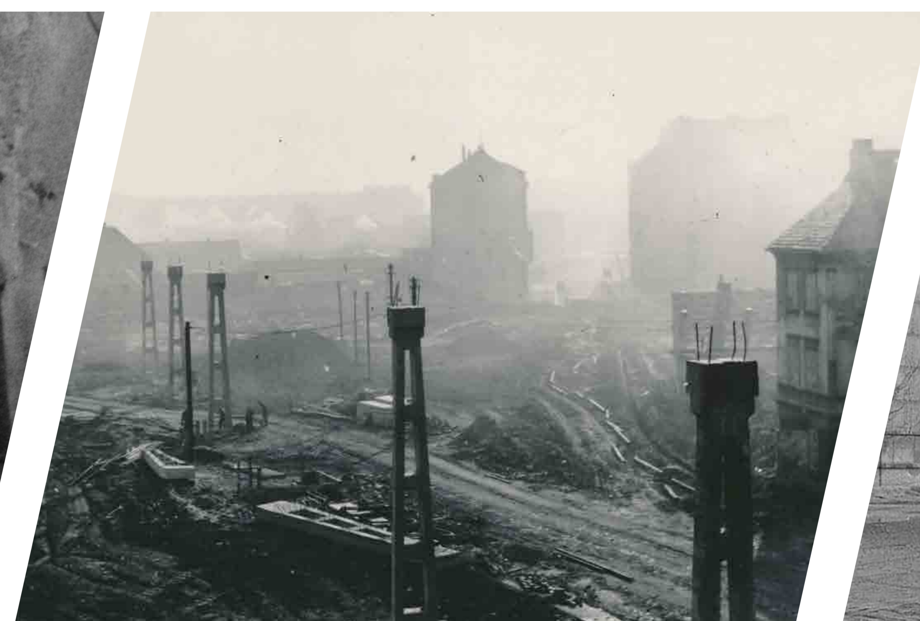
View from the construction site of the panel building towards V Závětří street, 1960.
