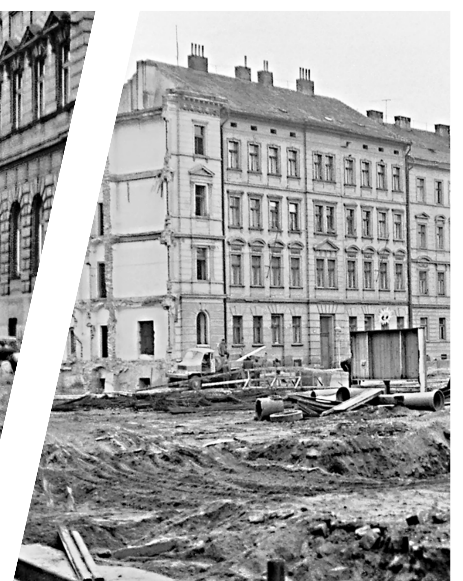
Demolition for new station, subway and highway 1978-1984.
