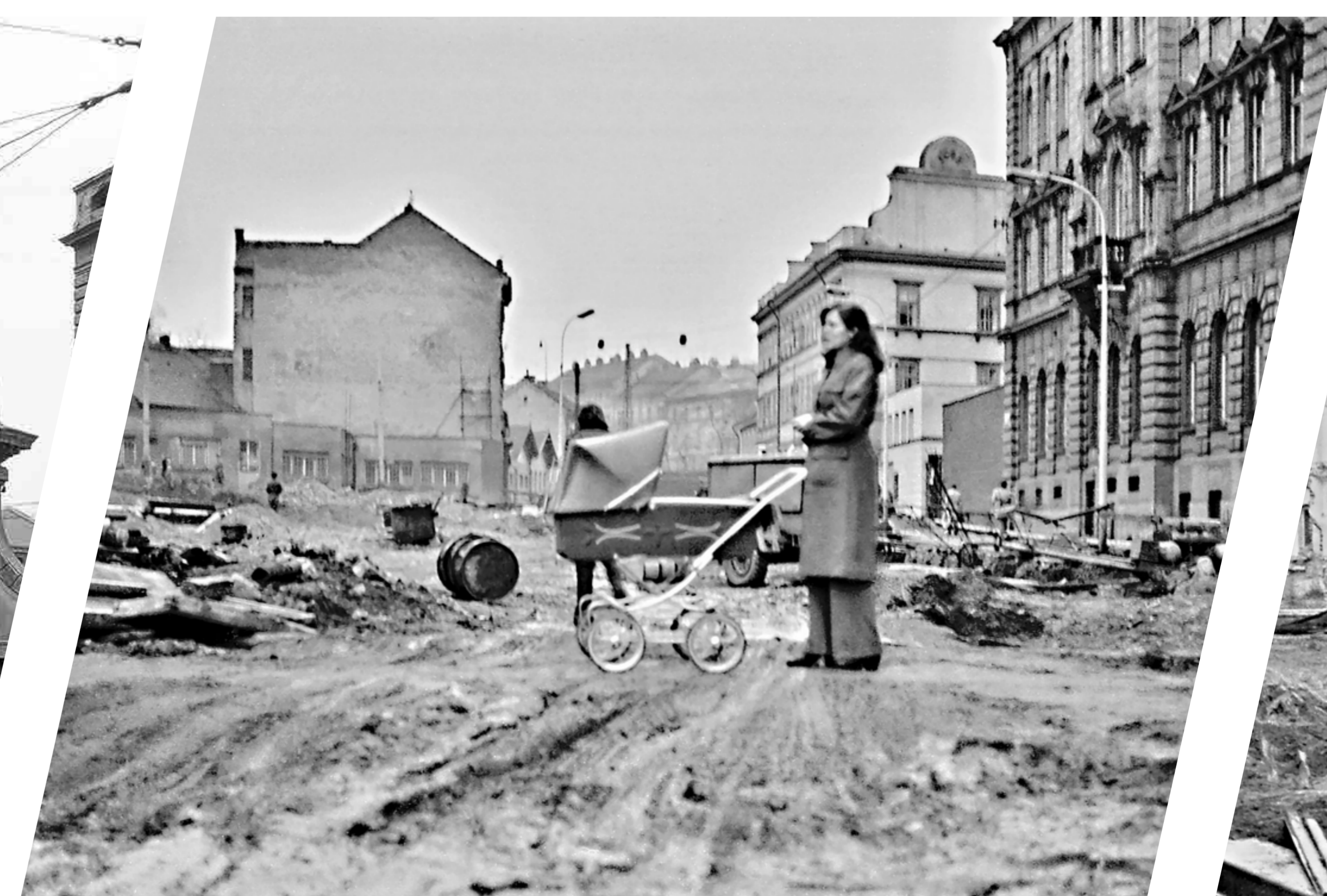
View along Partizánská street towards the Exhibition Grounds. On the right at the back, the existing house no. 218.
