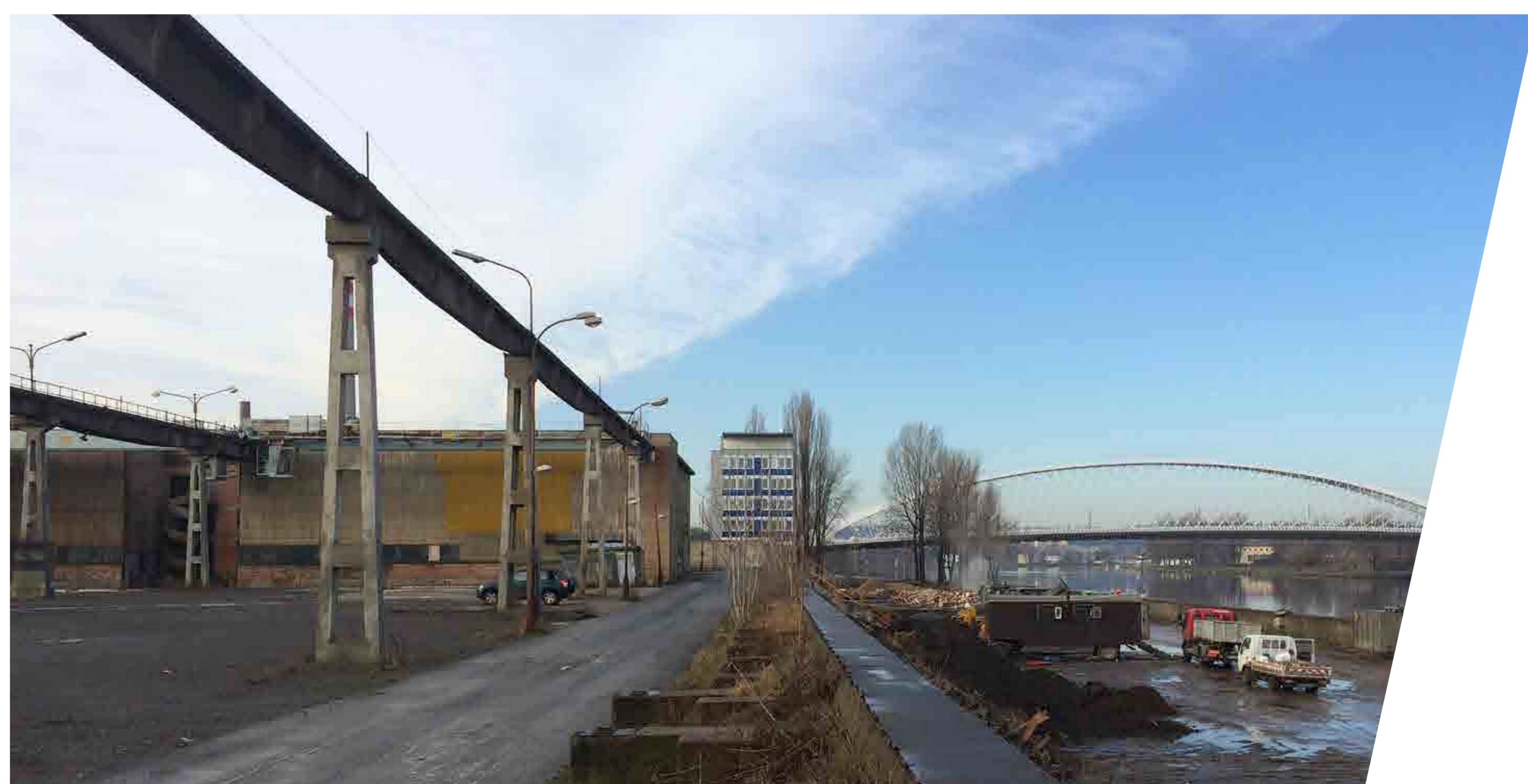
Crane tracks of overhead cranes for servicing the storage yard for finished products.
