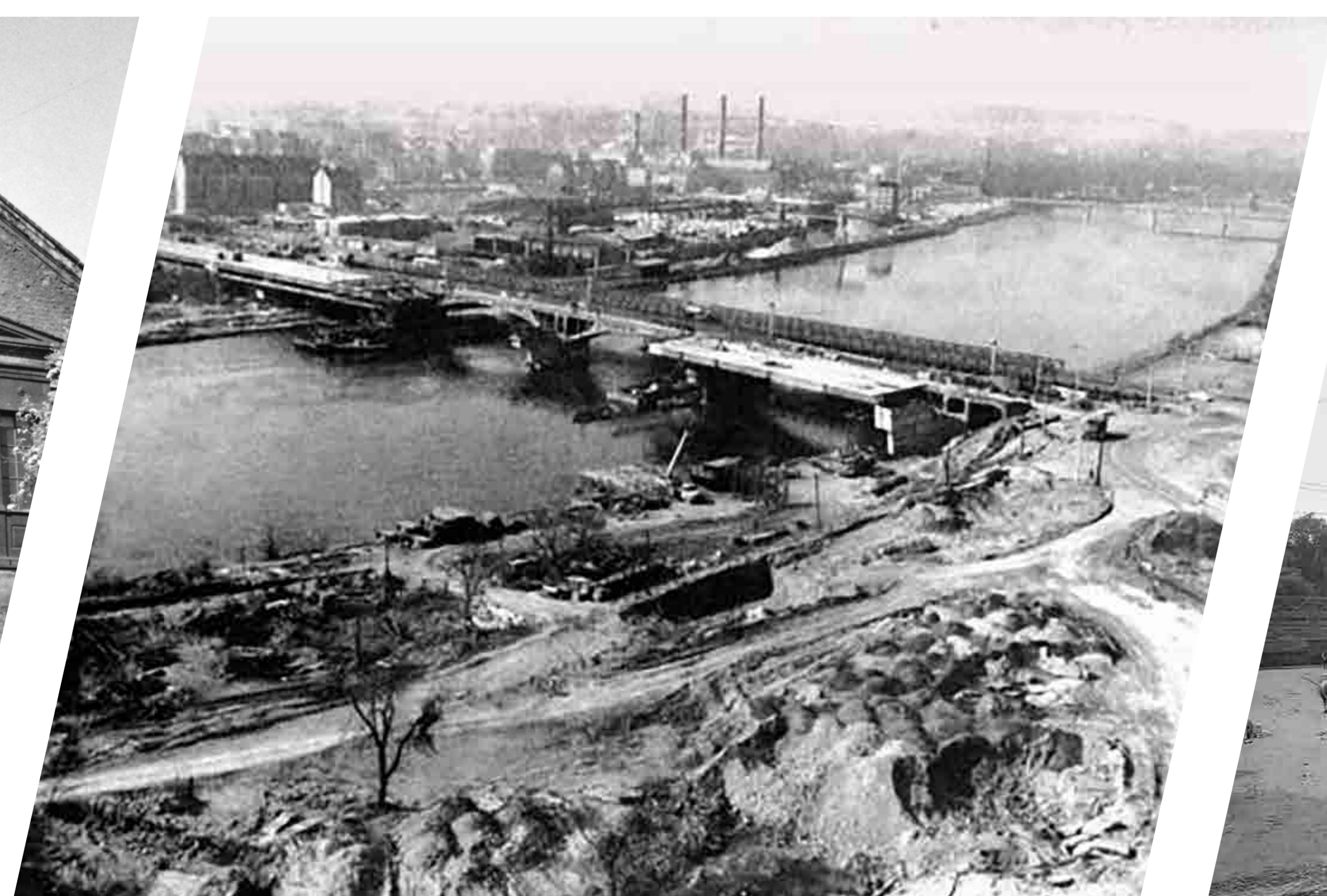
Construction of a new Barikádníků bridge on the site of the original Troja bridge.
