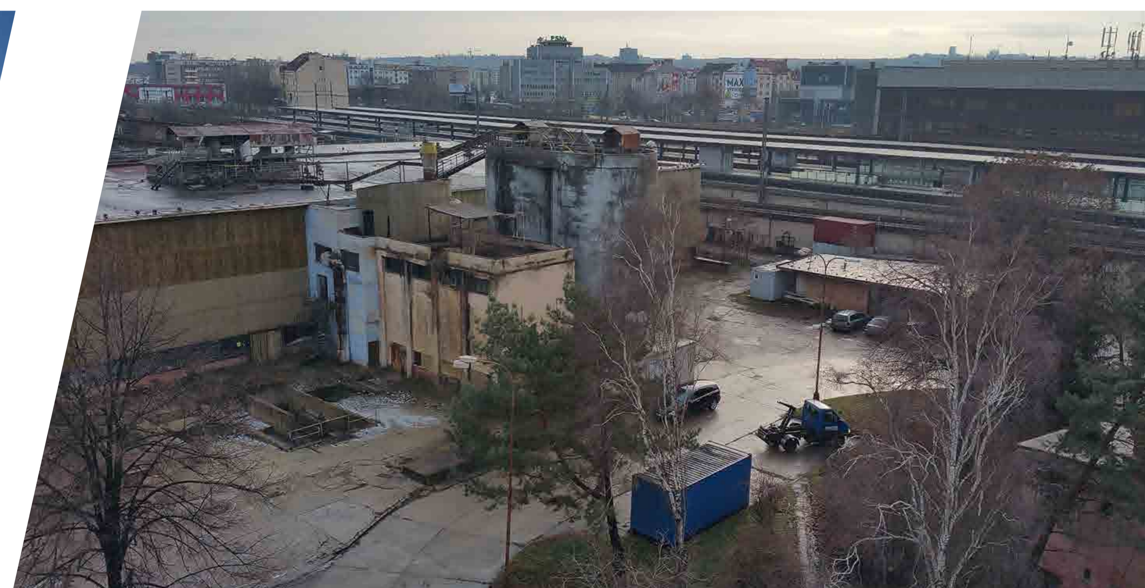
Production hall with cement silo, aggregate hopper and sludge pit.
