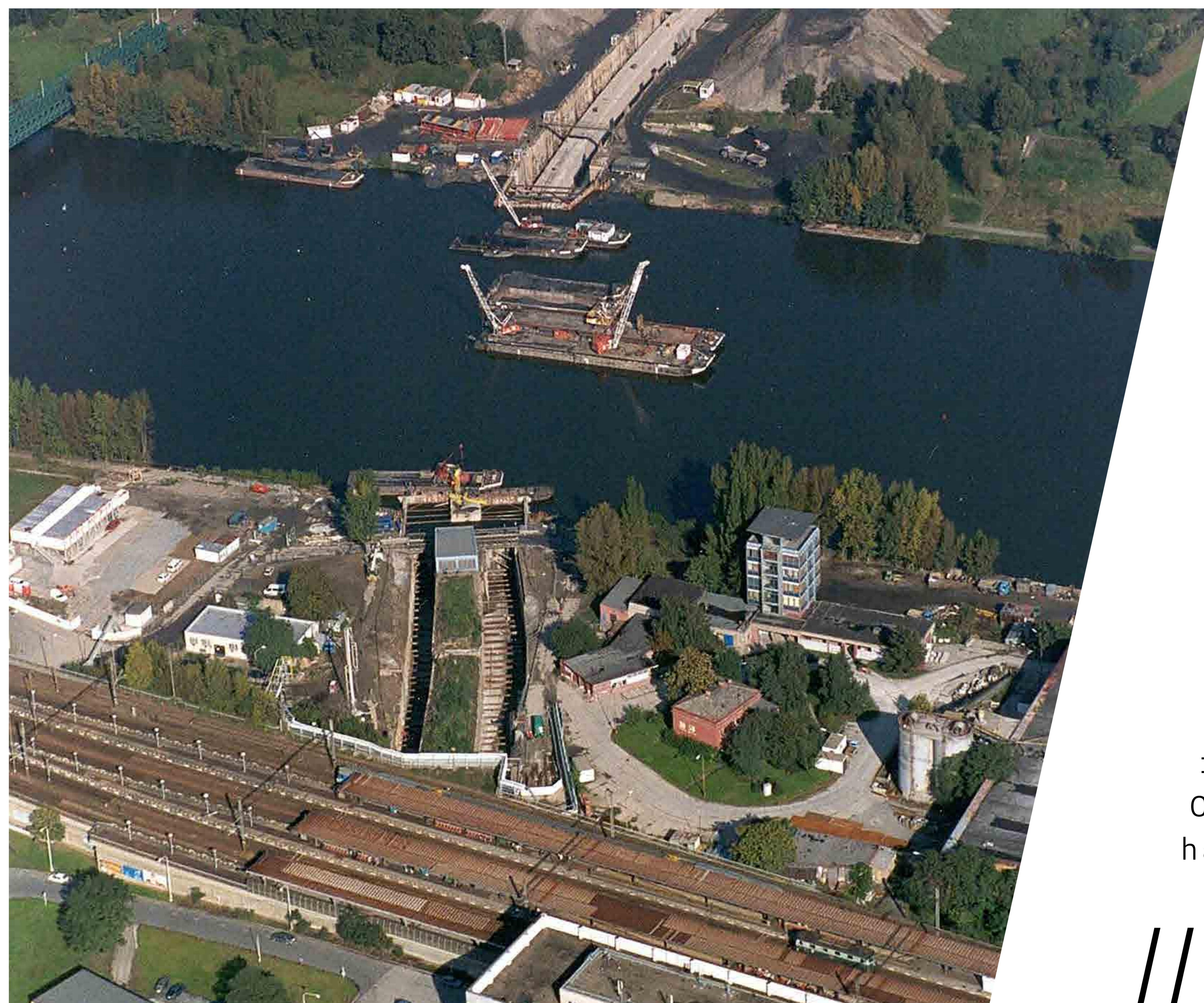
2003 - Construction of the metro in the direction of Ládví
